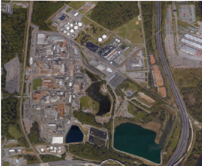
Aerial view of DuPont non-woven sheet manufacturing facility in Richmond, Virginia.
